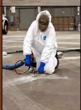
"SPF is an ideal product for void filling and concrete lifting," says Morgan. "We use the specially formulated, dense foam system made by one of the U.S.'s oldest and most trusted foam houses, NCFI Polyurethanes. We removed the asphalt and drilled small holes in the slabs, pumped the two-part TerraThane™ foam into the holes to fill the voids—some larger than 36"—then raised the slabs to level."
